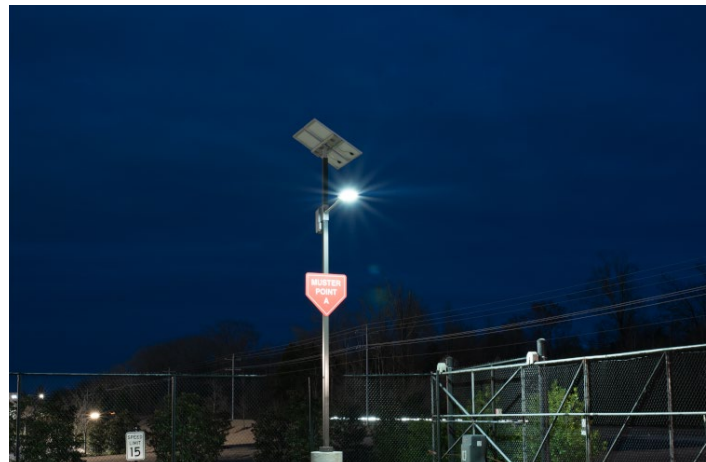
12380 Kirk Rd, Olive Branch, MS Parking Lot Lighting Project
