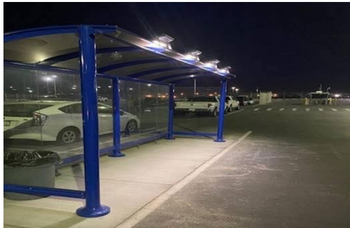
San Francisco International Airport California, USA Bus Shelter Lighting Project
